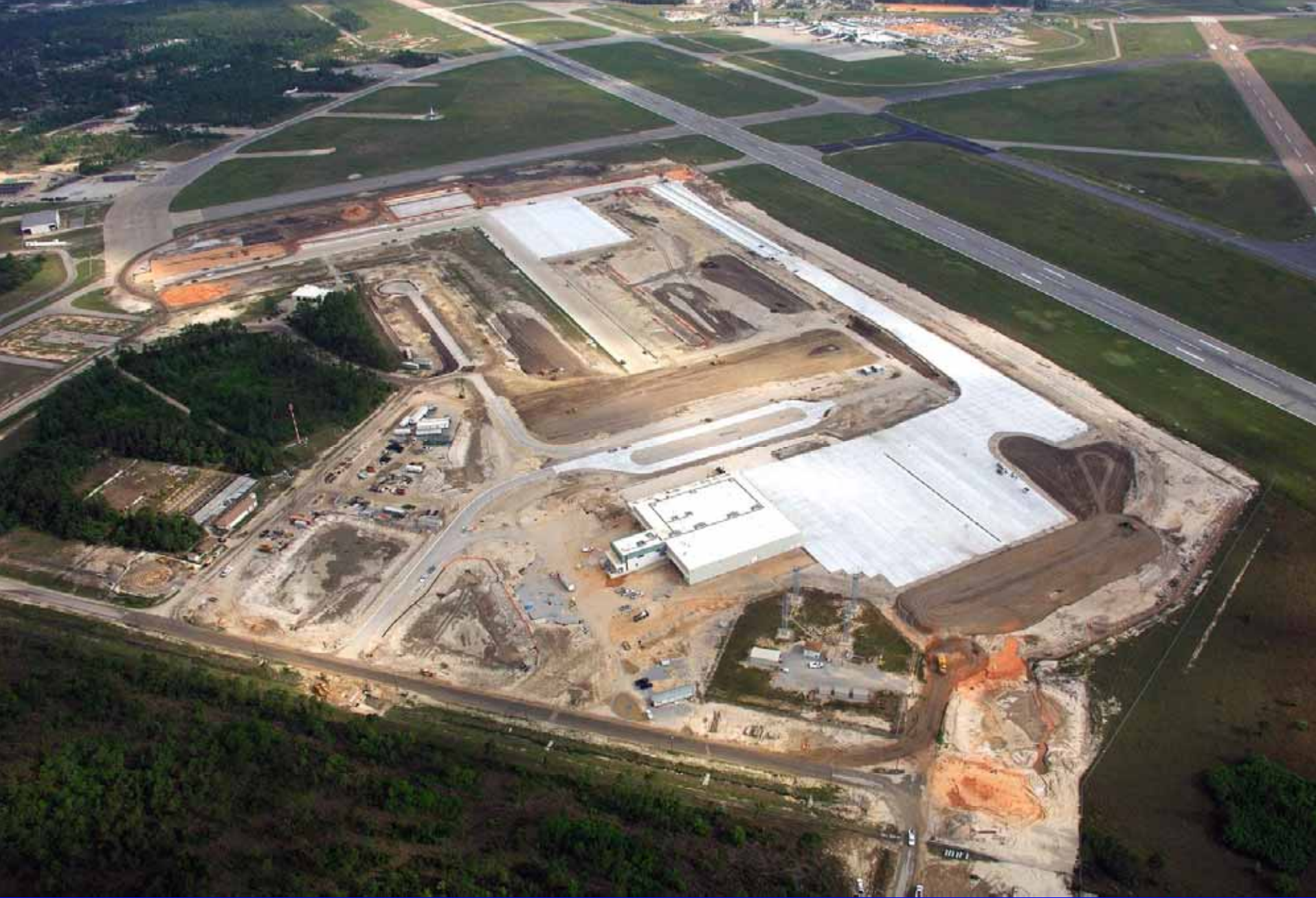
Gulfport-Biloxi International Airport Air Cargo Facility
