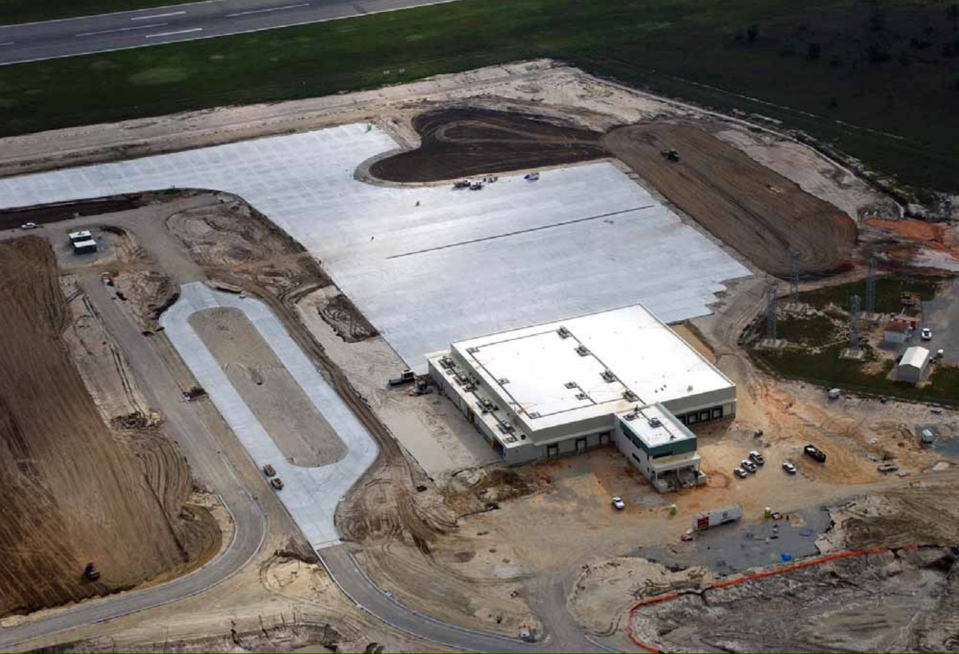
Gulfport-Biloxi International Airport Air Cargo Facility
