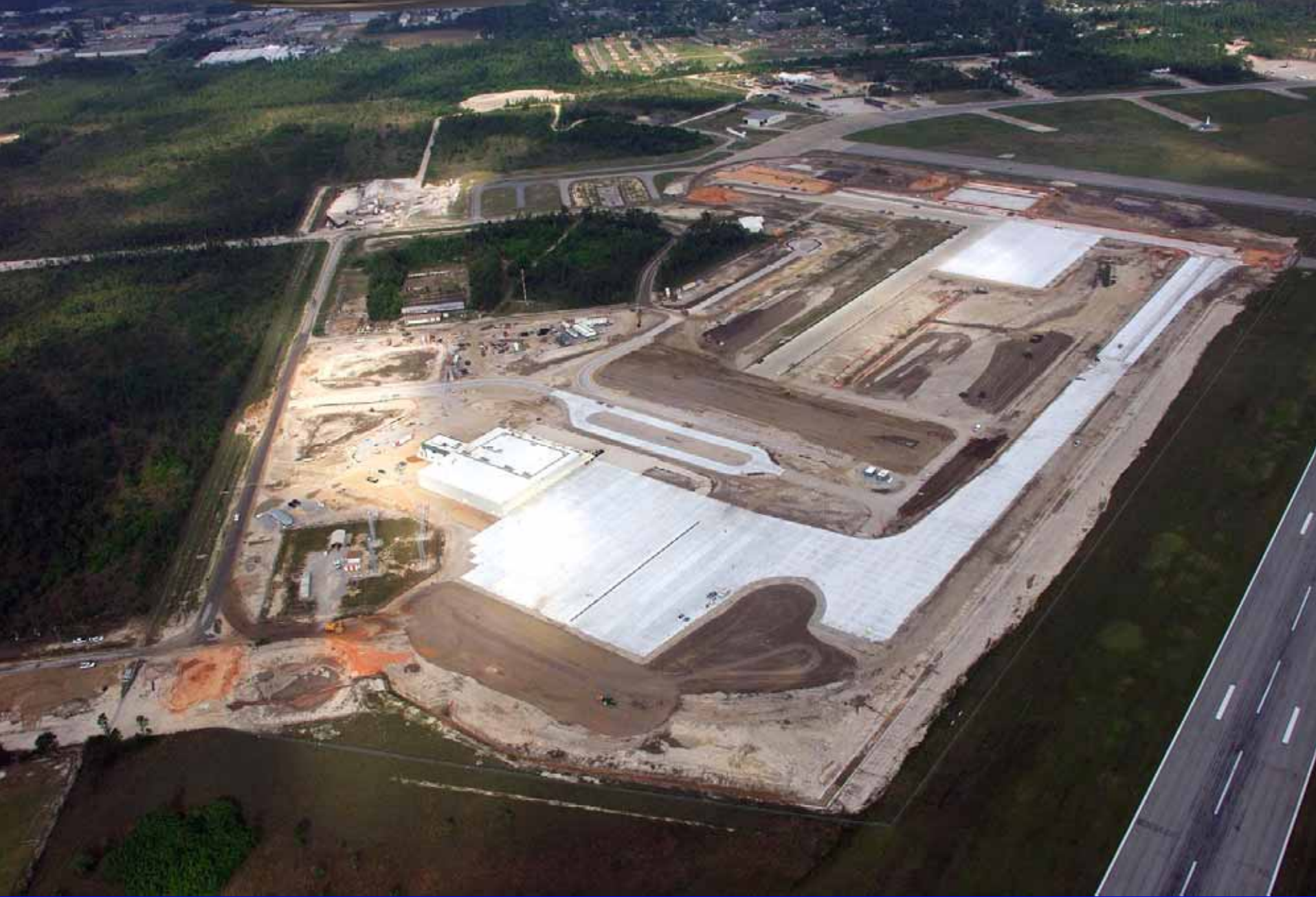
Gulfport-Biloxi International Airport Air Cargo Facility
